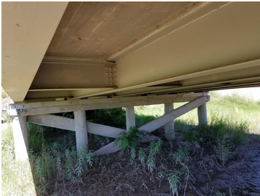
Underside of bridge (typ.) looking North
