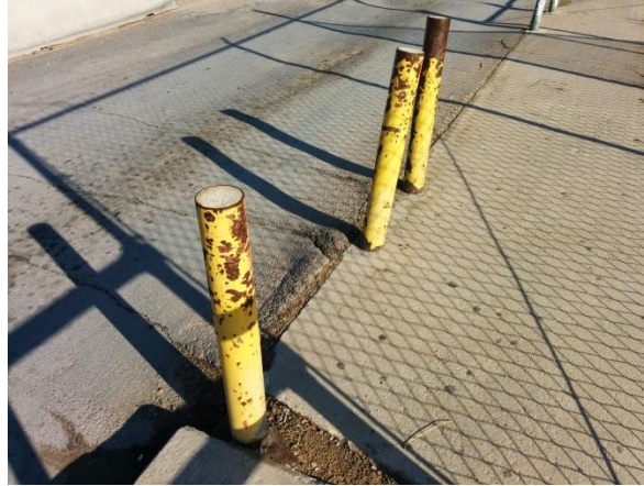
Concrete filled bollards
