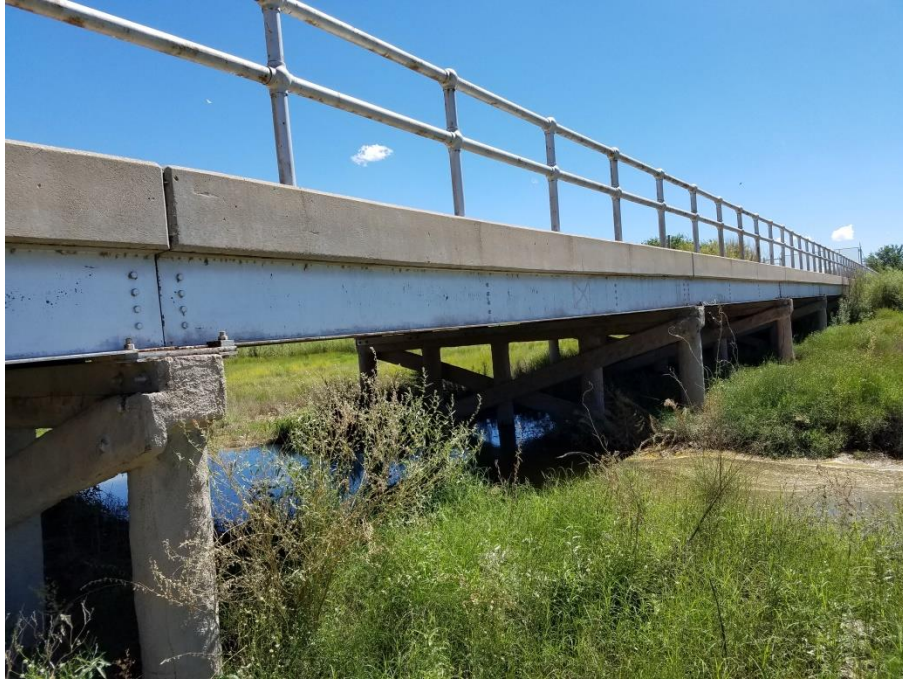
West side of the bridge, looking south.
