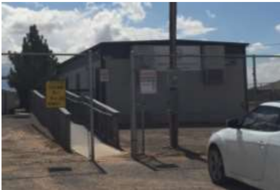
View of Exterior Door
