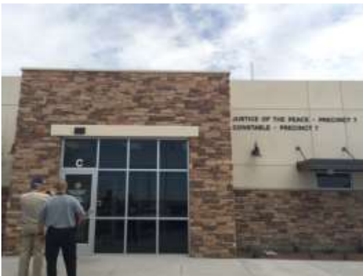
View of Exterior Door
