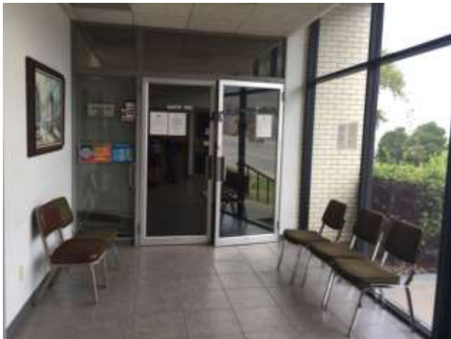
View of Exterior Door
