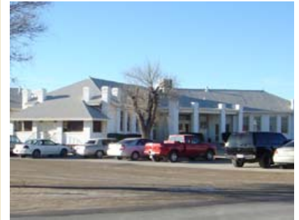
Socorro Administrative Complex
