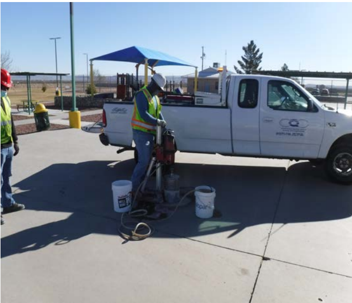
PHOTO NO. 7: General view of our coring operation at vertical boring B-3.
