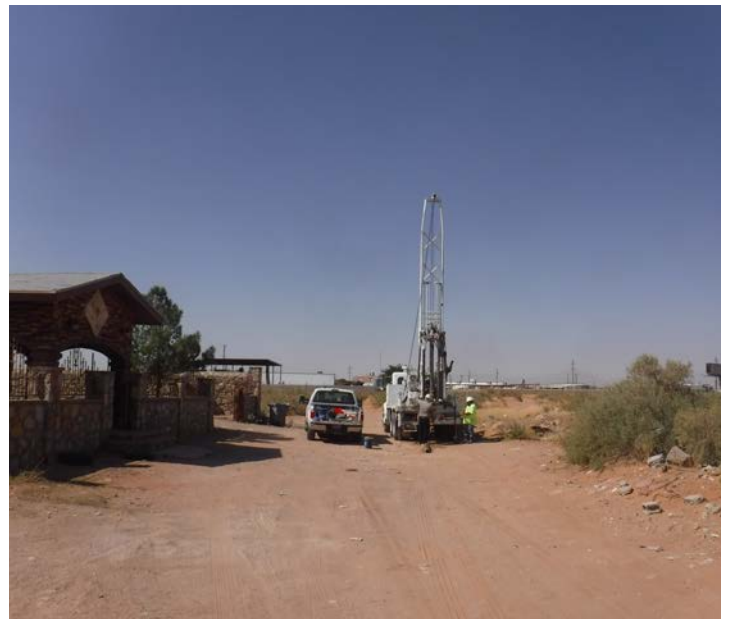
PHOTO NO. 8: General view of our subsurface soil drilling operations at vertical boring B-1.
