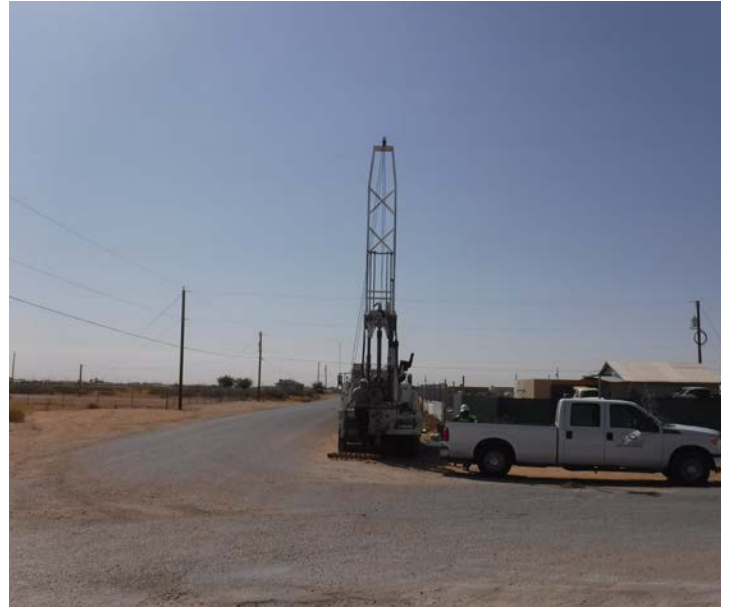
PHOTO NO. 10: General view of our subsurface soil drilling operations at vertical boring B-4.
