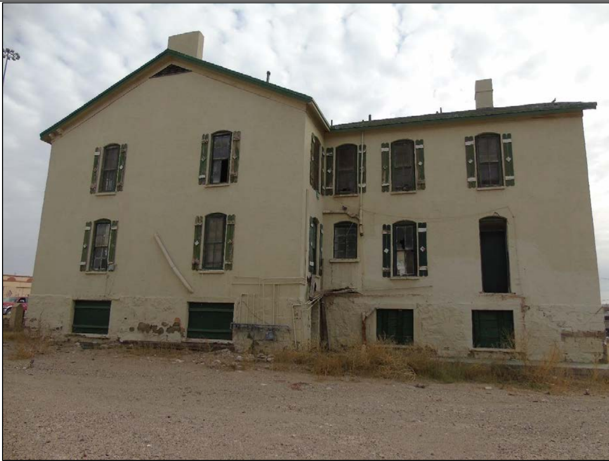
1836 West Paisano. North façade, camera facing South.
