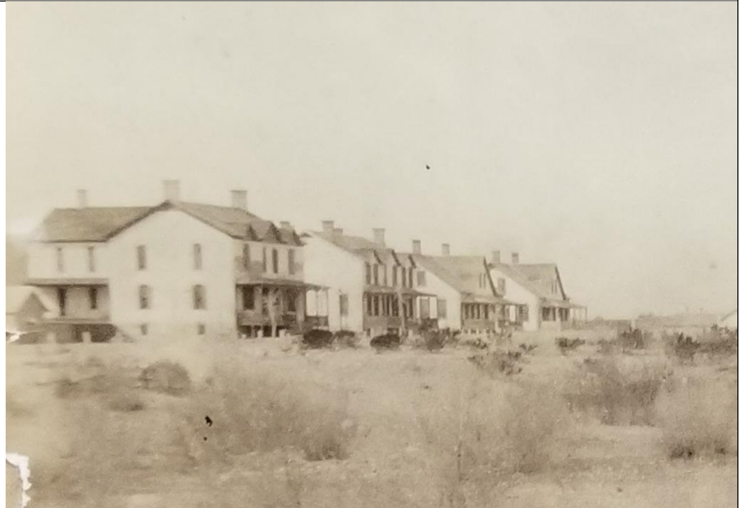
1844 West Paisano is second building on the left. El Paso Public Library - Aultman collection, 1885.
