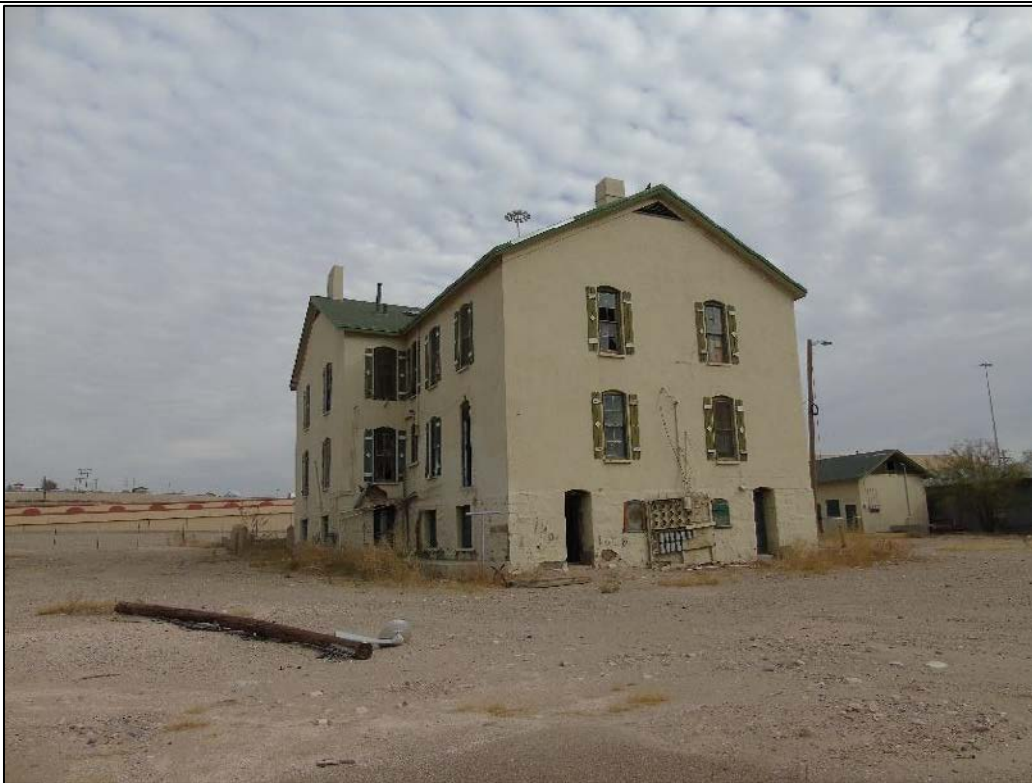
1836 West Paisano. Rear facade, camera facing Southeast.
