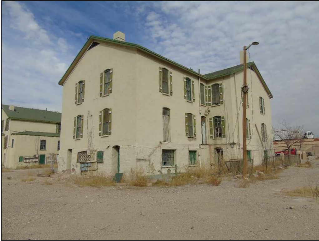
1836 West Paisano. Southwest. façade, camera facing Northeast, 1844 W Paisano is visible to the left.
