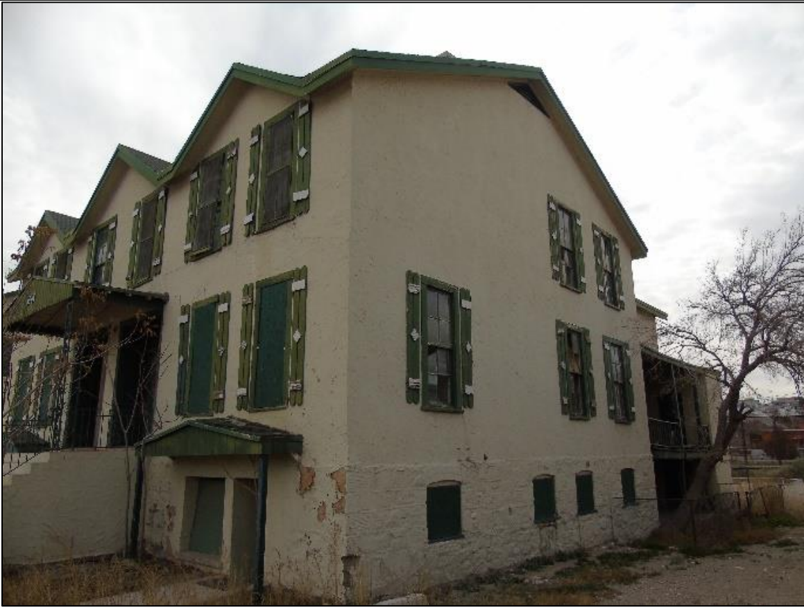
1844 West Paisano. Northeast façade, camera facing southwest.
