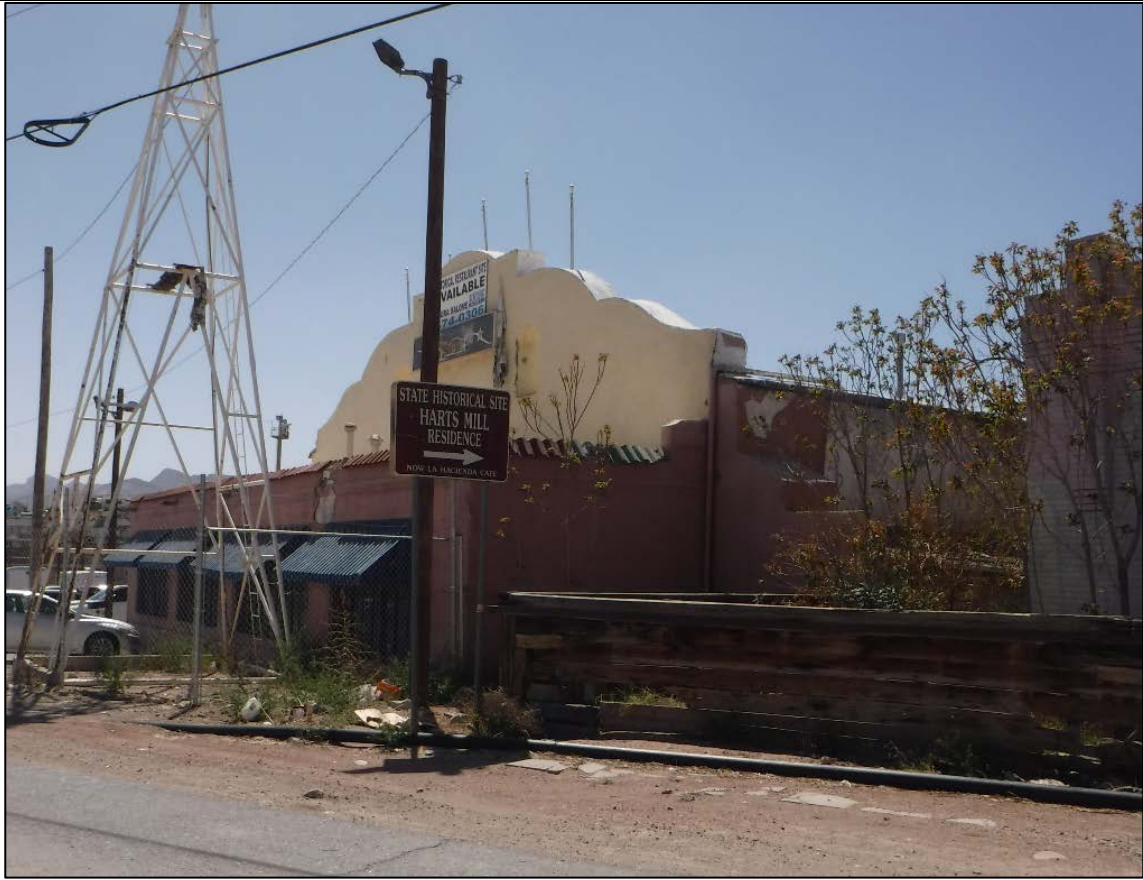
1720 West Paisano, camera facing southwest.
