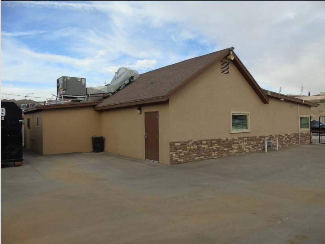
1932 West Paisano. West facade, camera facing northwest.
