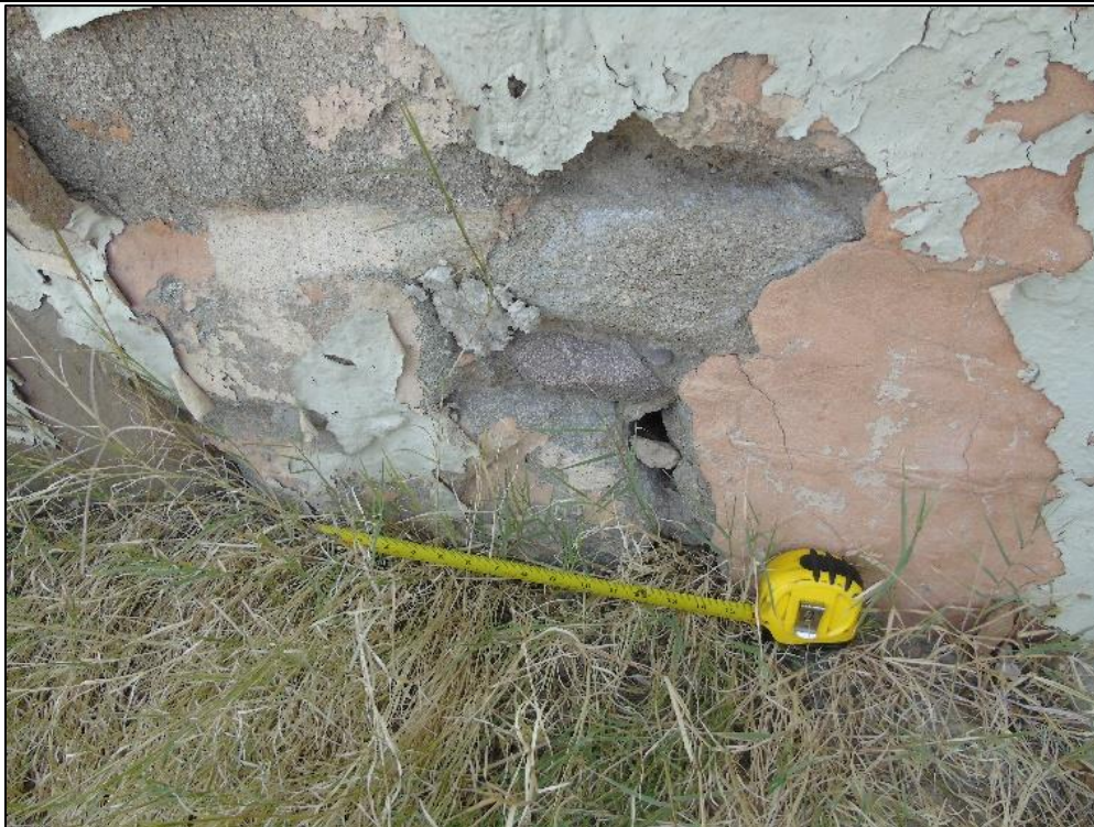
1844 West Paisano. Foundation detail, southeast corner.
