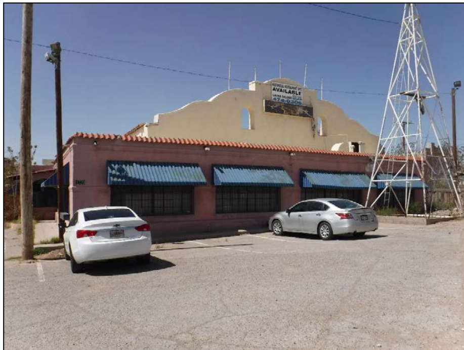
1720 West Paisano. Front facade, camera facing northwest.
