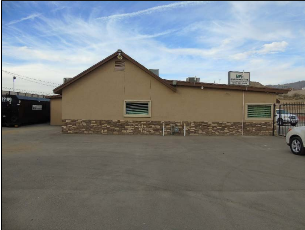
1932 West Paisano. South façade, camera facing north.
