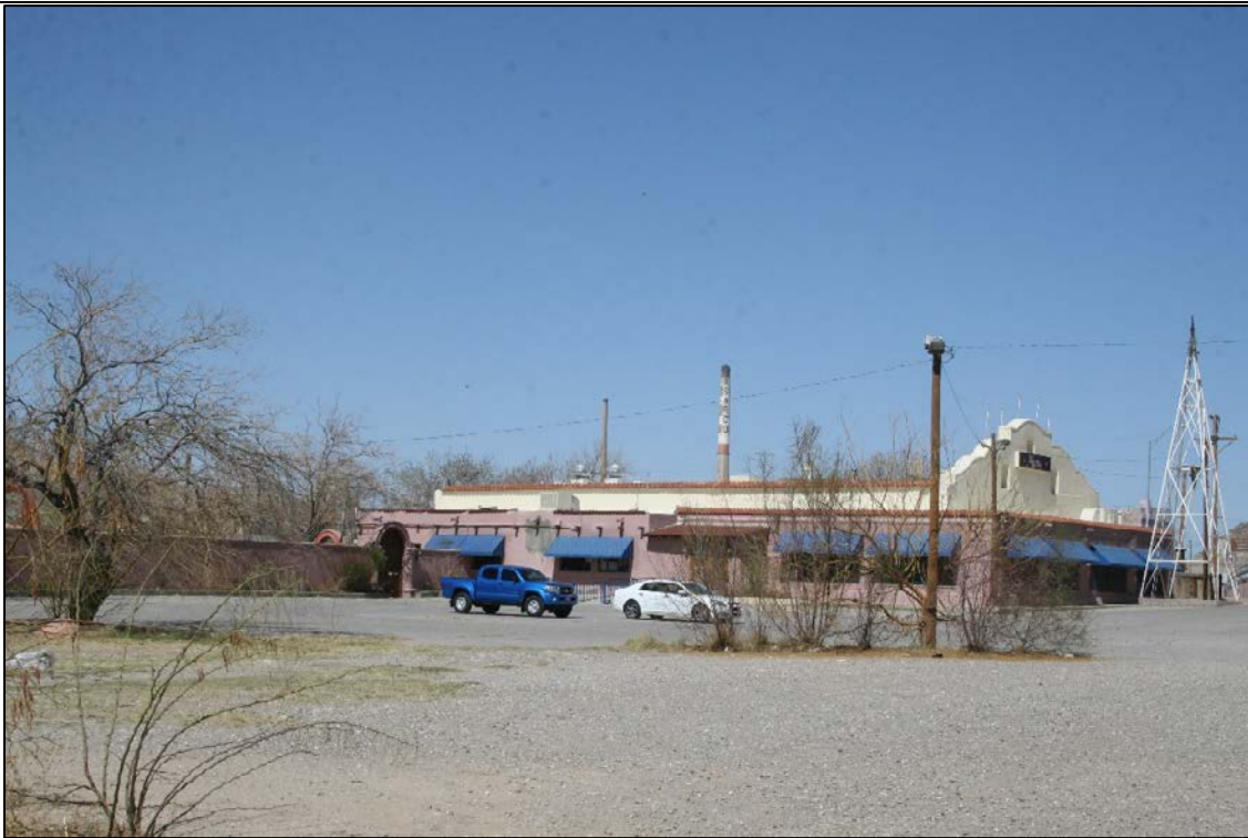
1720 West Paisano. Southeast façade, camera facing Northwest.
