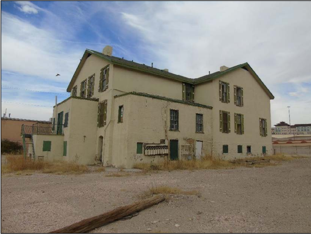
1844 West Paisano. Southwest façade, camera facing Northeast.
