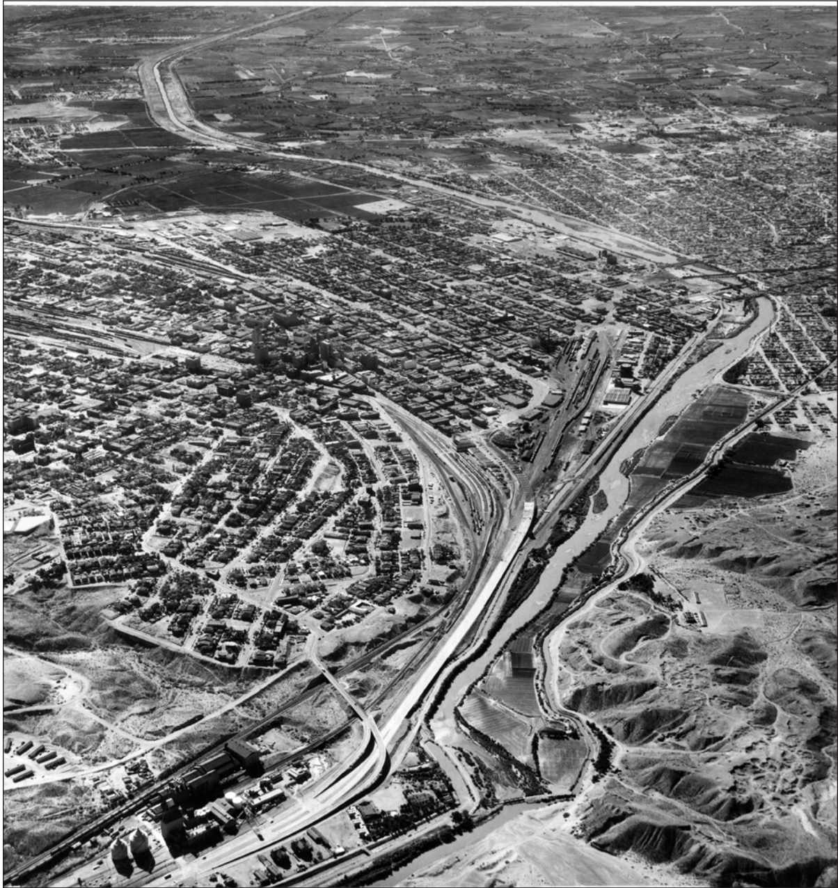
Figure 4-31. A 1955 bird's eye aerial photo looking southeast along the Rio Grande. Agricultural fields of Mexico and Texas can be seen at the top of the photograph and along the Acequia Madre. The Hart's Mill area is at the bottom (courtesy of TxDOT).
