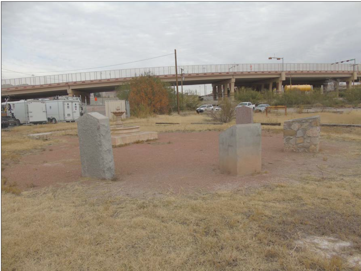
Figure 4-45. View from the former Hart's Mill looking toward the Yandell Street Bridge that splits the Oñate Crossing landscape on the American side and cuts off access to the remaining features from elsewhere in El Paso.
