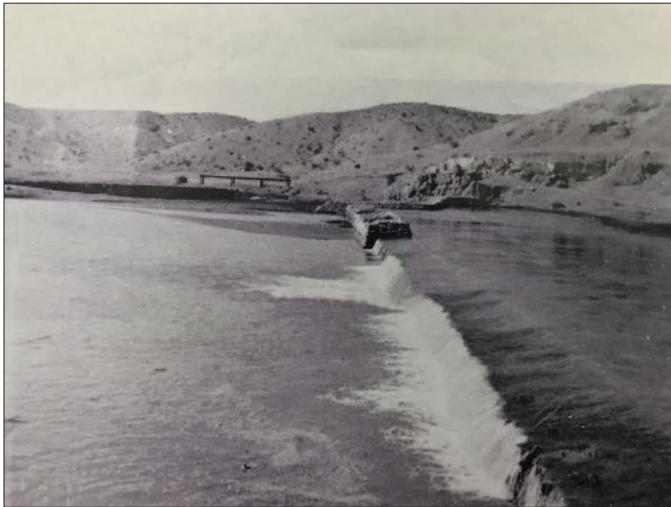
Figure 3-12. 1934 Photograph of the 1907 International Dam at Hart's Mill (courtesy of IBWC).
