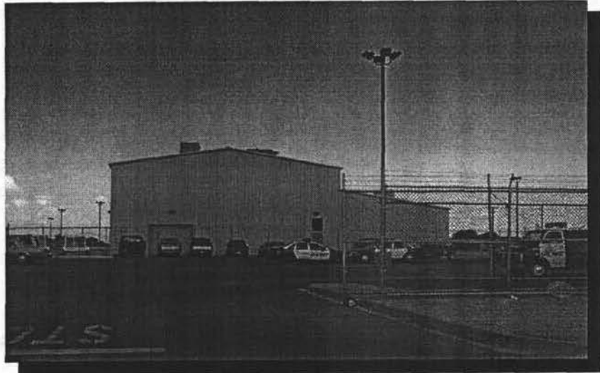
Sheriff Substation in East El Paso next to the Leo Samaniego Law Enforcement Complex (Jail Annex)
