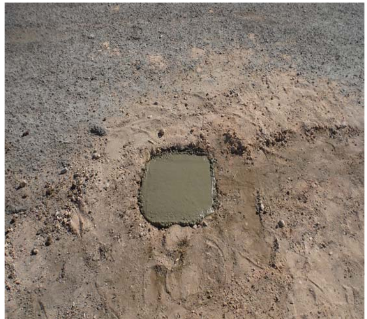
PHOTO NO. 8: General view of a soil boring location patched with 3,000 psi concrete along Montana Avenue alignment.
