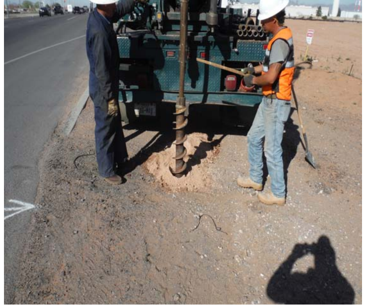
PHOTO NO. 6: View of the drilling activity at soil boring location B-30 and existing site conditions.
