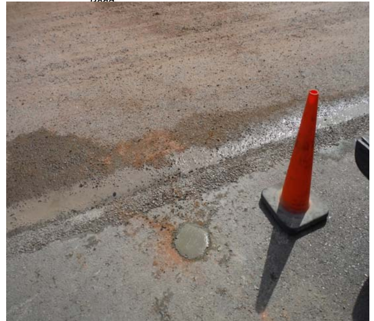
PHOTO NO. 12: General view of a soil boring location patched with 3,000 psi concrete along Square Dance Road.
