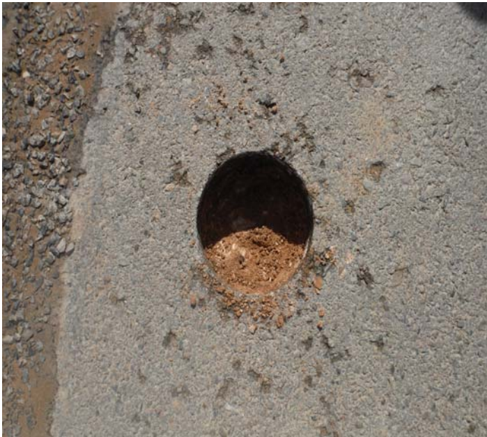
PHOTO NO. 11: View of the subsurface soils after being hydro-compacted and ready for the concrete patch along Square Dance Road.
